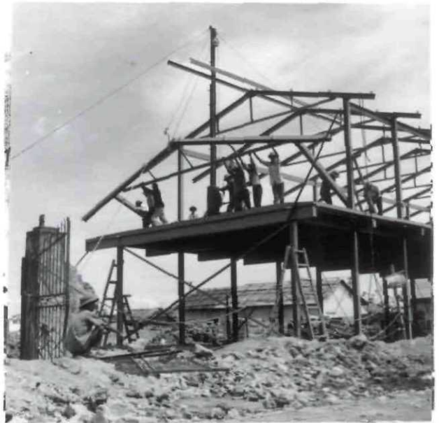
Above and below: The last frame on first floor lifted by the ginpole and bolted into position.
