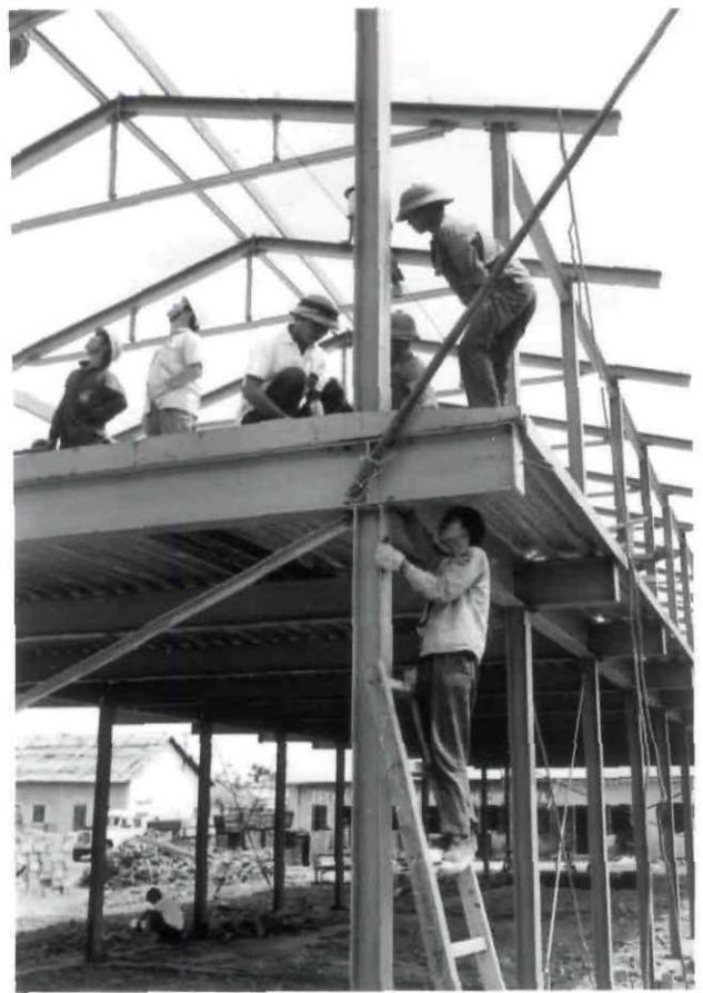
Above and below: The last frame on first floor lifted by the ginpole and bolted into position.
